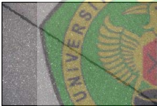
Gambar 2.7 Diagonal Cracks
